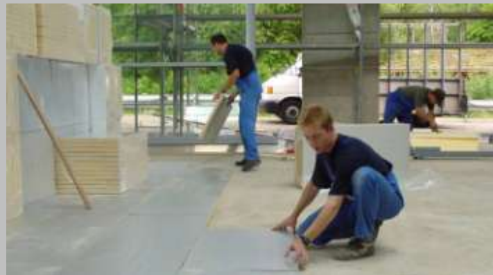
PU insulation board in floors
